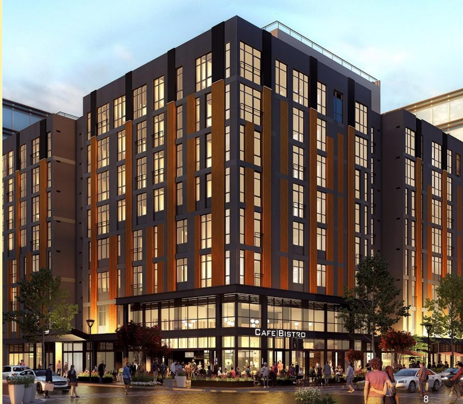
Conversion of Peace Corps offices into Elle apartments, delivered in 2024
