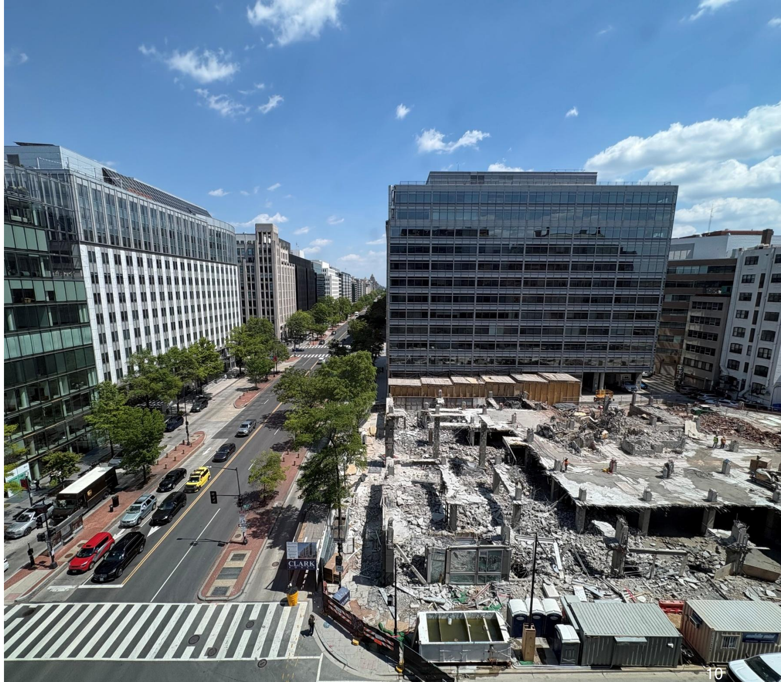
Office to residential redevelopment underway along K Street
